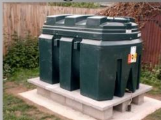
Oil Tank Installation
