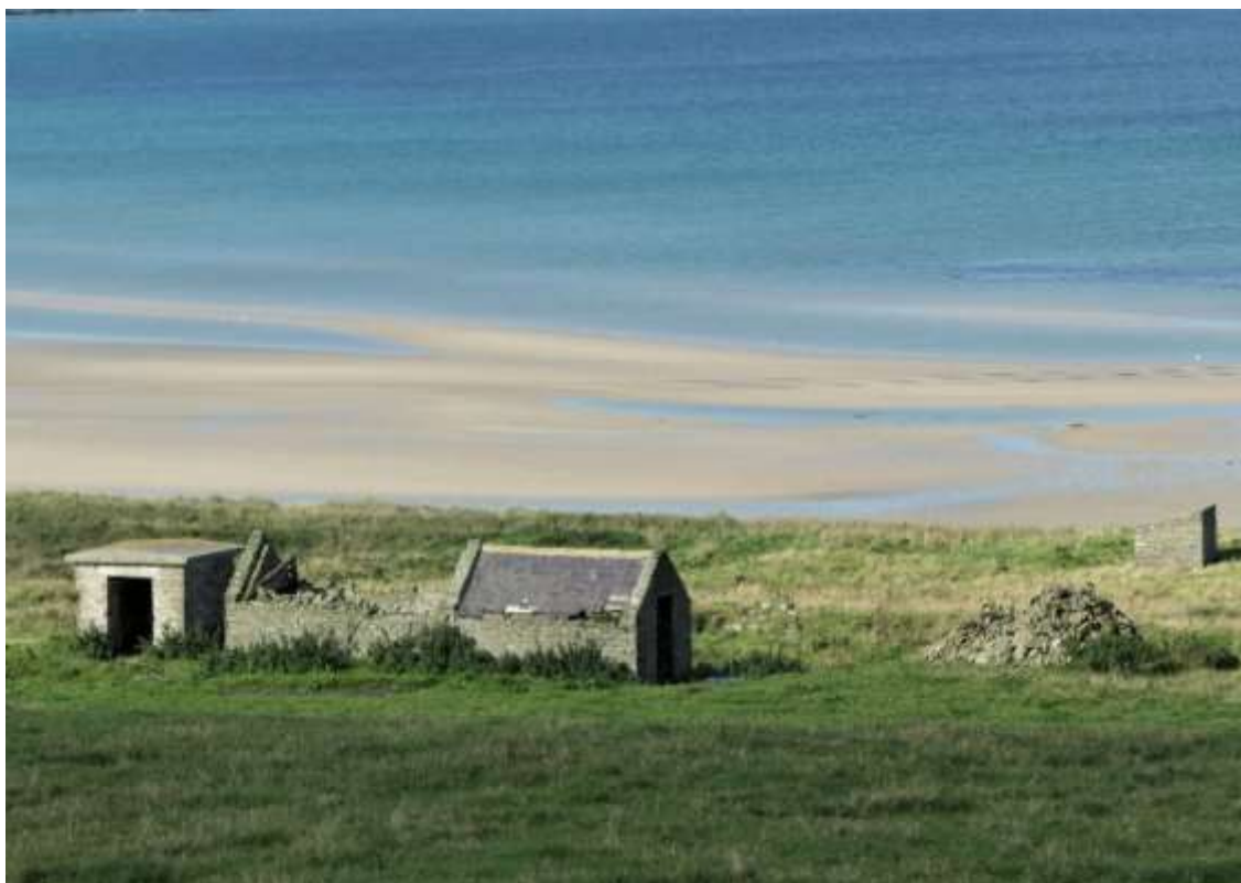
This is what remains of the Stronsay rifle range, where servicemen practised their shooting skills
