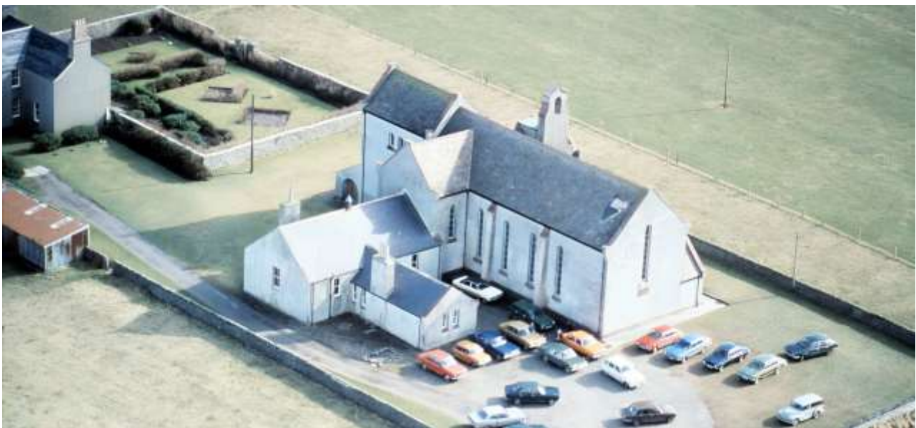
An aerial view of the church showing storm damage to the roof
