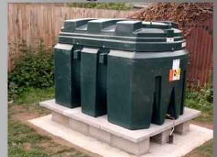
Oil Tank Installation
