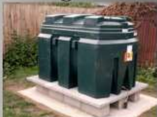
Oil Tank Installation
