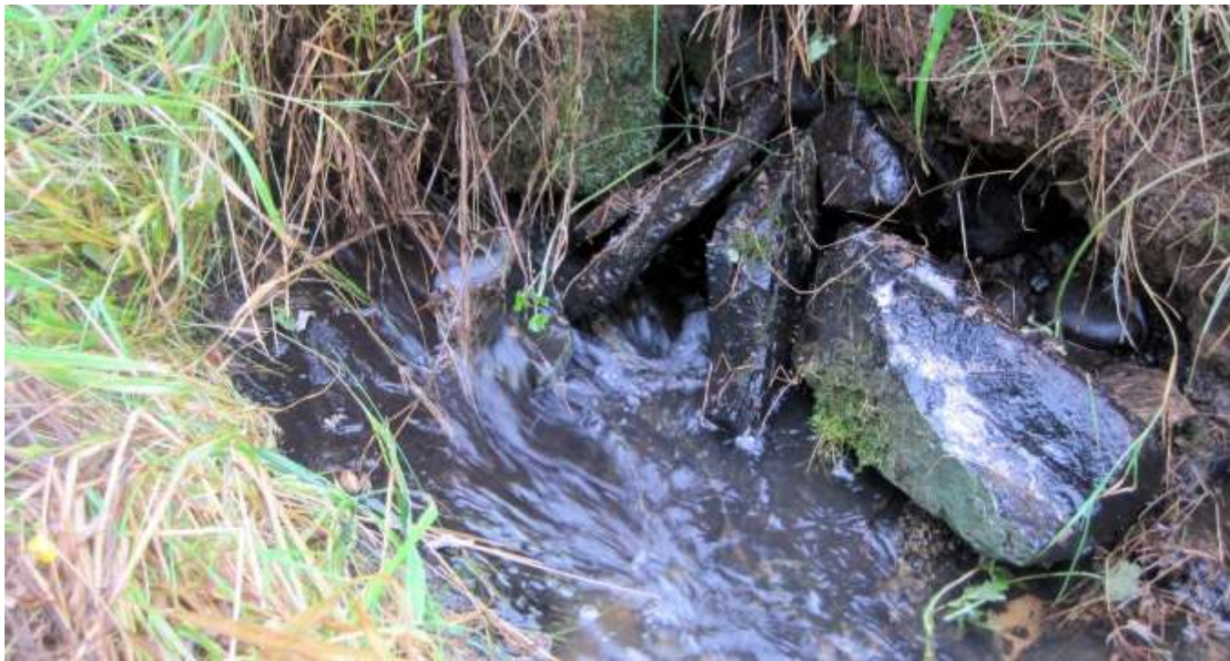
The inverted ‘V’ shape of a coupled drain, still successfully draining the land and feeding water into a ditch after more than 150 years.
