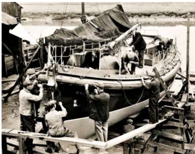
The Edward Z Dresden on the slip undergoing repair. This included filling up the bullet holes, smoothing out the scrapes and scuffs and giving her a new coat of paint after her rescue mission to assist with the Dunkirk evacuation in May 1940.
