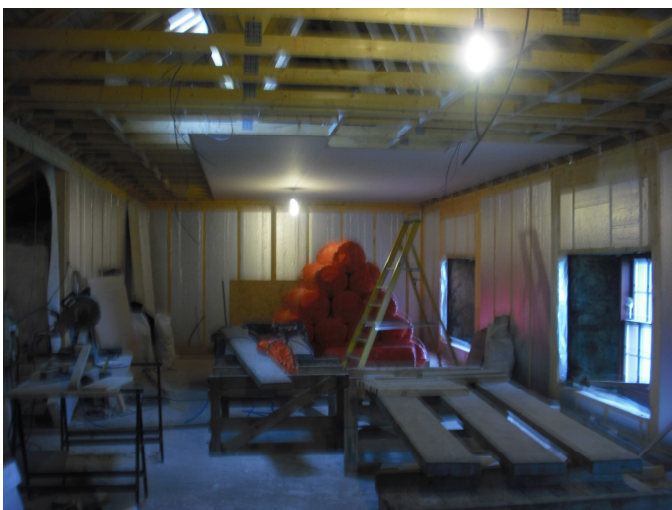
Top floor ceiling partly plaster-boarded
